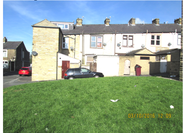
looking towards rear of March St houses
