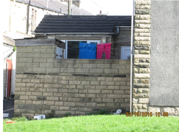
side/ rear of 8 Clive Street
